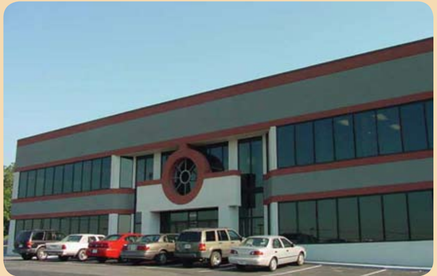
Free Will Baptist National Office Building - Antioch, TN
